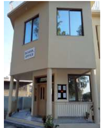
Front Office Entrance of Tarnol
